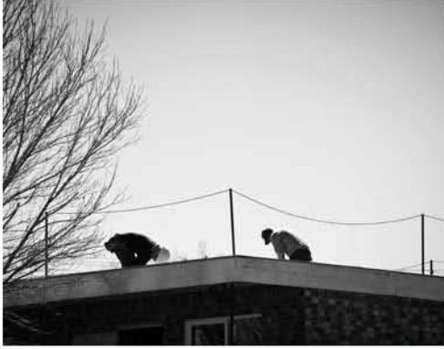
- Workers repair the roof of La Hacienda Apartments in Belen.
