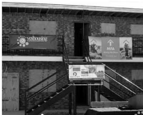
- La Hacienda Apartments before renovation began.
